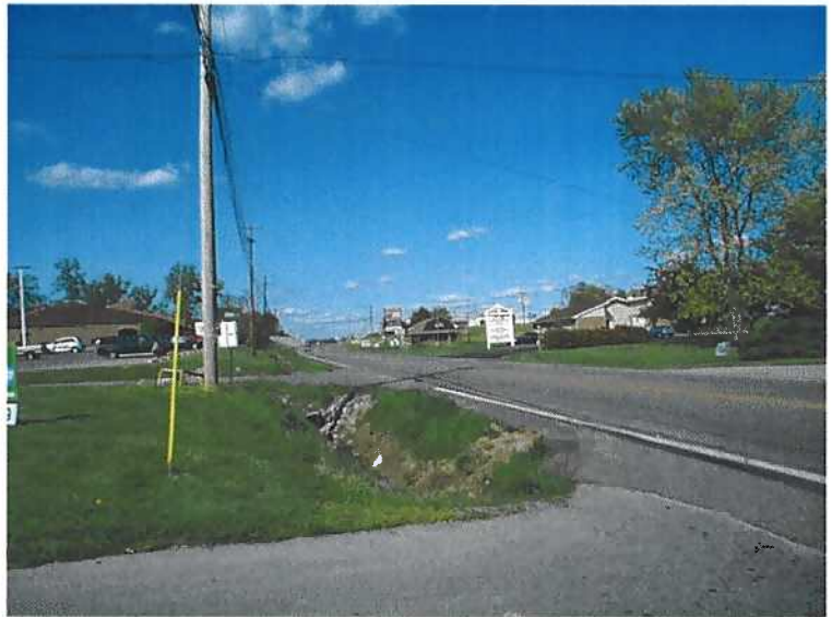
US 60 typical with residential and commercial property
